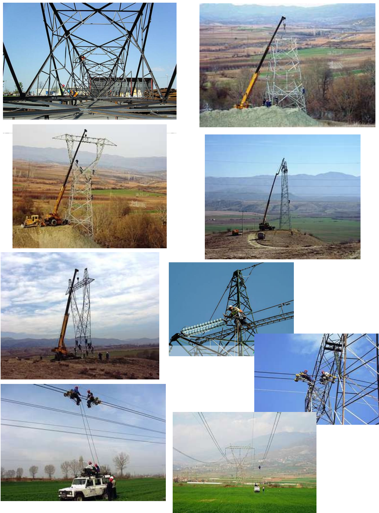
Figure 3-3 — Construction and installation of a single circuit 400 kV transmission line infrastructure
