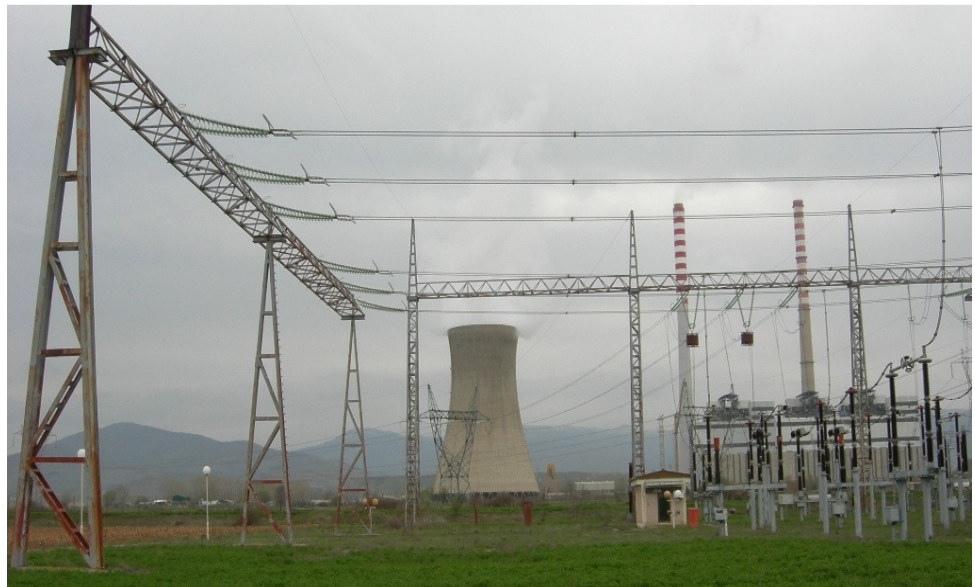
Figure 3-7 — Spare bay in the existing substation Bitola 2 which will accommodate the proposed transmission line
